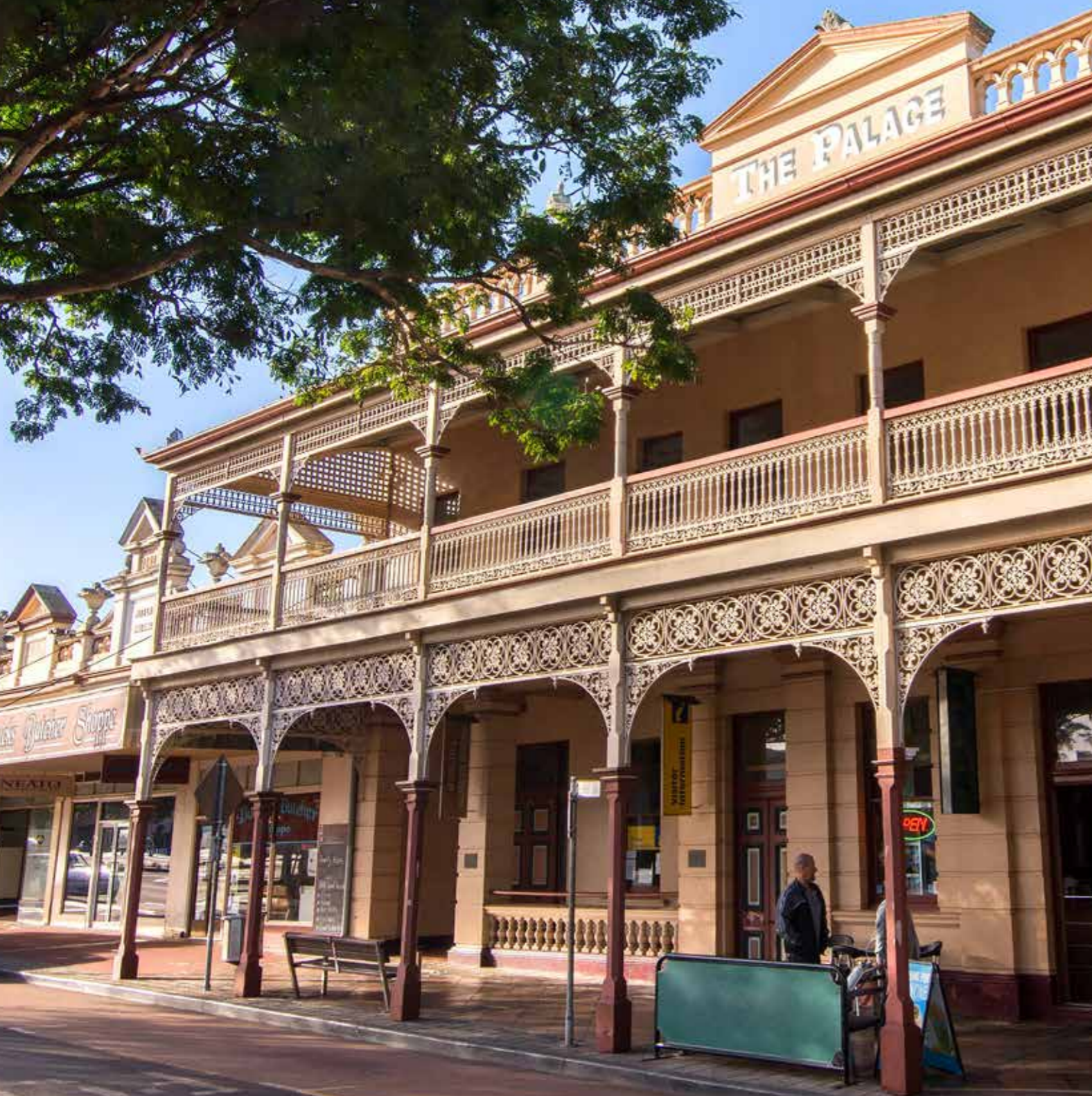
The Palace Building, Childers
