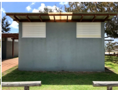
Building 1: Stage 2 wall
