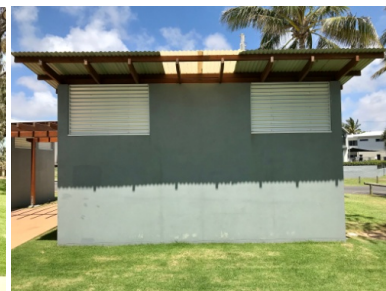
Building 2: Stage 2 wall
