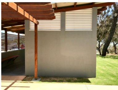
Building 2: Stage 1 wall
