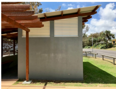
Building 1: Stage 1 wall
