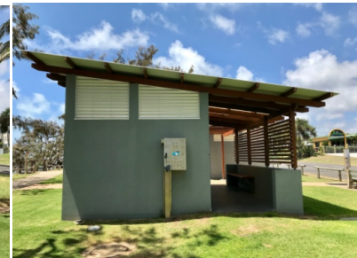
Building 2: Stage 3 wall
