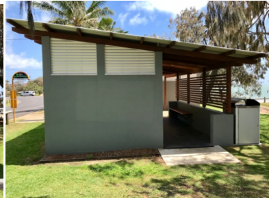
Building 1: Stage 3 wall
